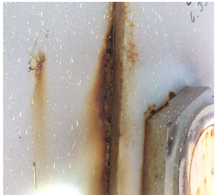
PHOTO 2 Description Corrosion with pack rust to pin and hanger assemblies.
