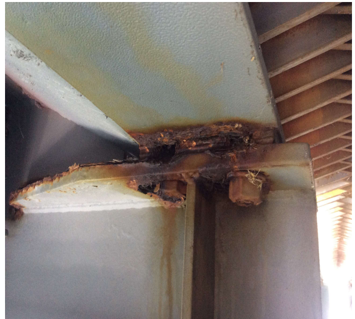
PHOTO 2 Description Corrosion at stringer/finger joint connection.
