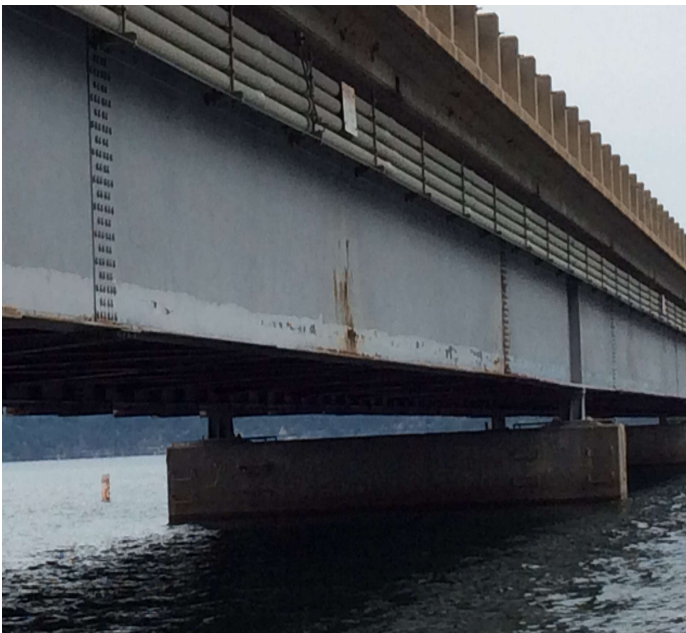
PHOTO 1 Description Span #2 minor section loss to bottom flange and lower 1/2 of web in girder #1
