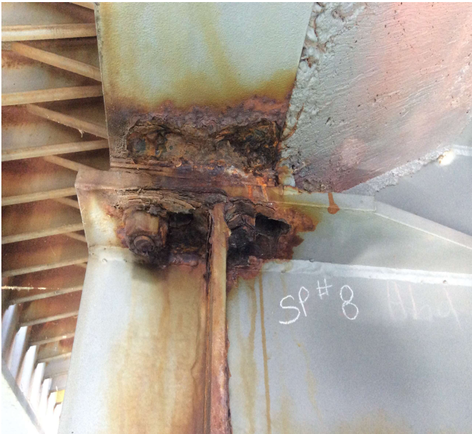
PHOTO 4 Description Corrosion at stringer / floorbeam connection.
