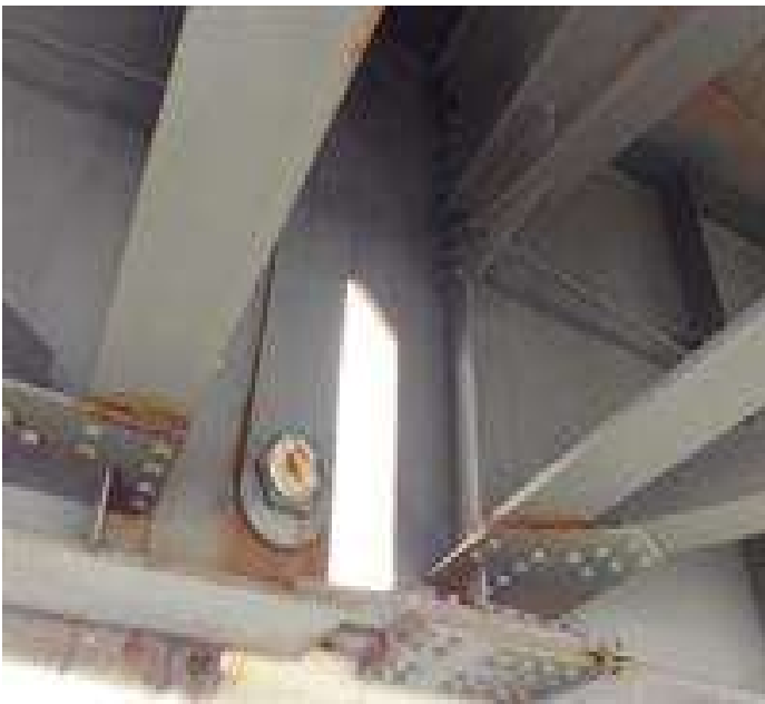
PHOTO 4 Description Span #8 Lower Hanger Assembly
