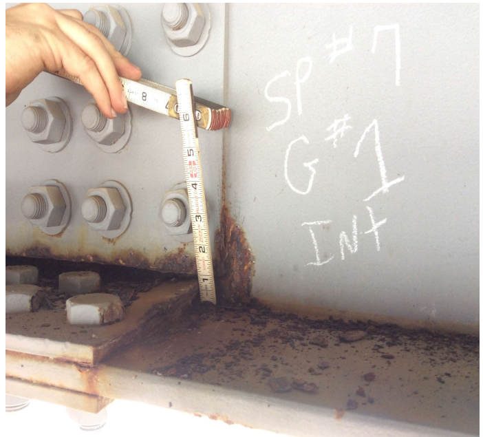
PHOTO 2 Description Pack rust with out-of-plane bending to connection plate.
