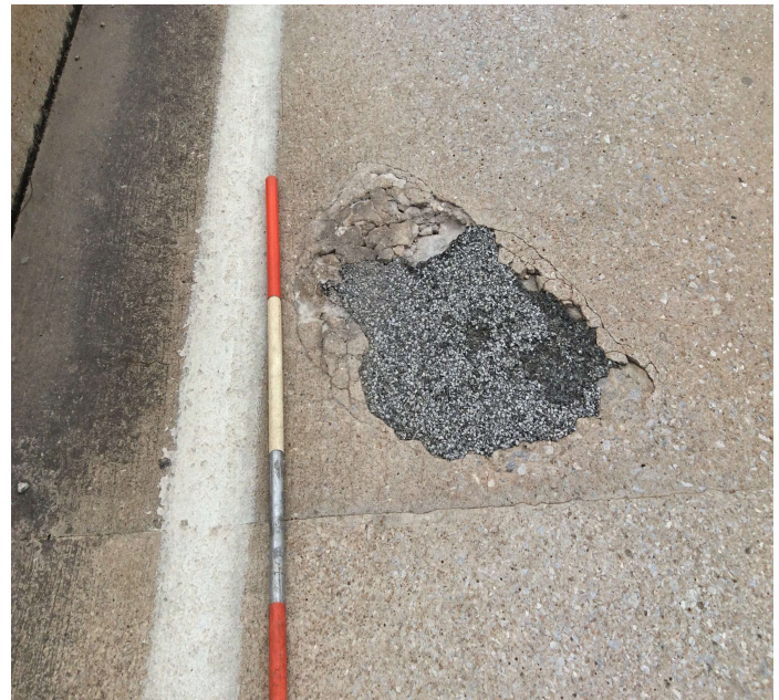
PHOTO 5 Description Deck spalling typical.
