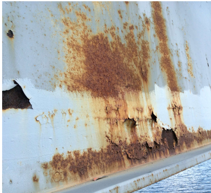
PHOTO 3 Description Span #5, girder #1, paint failure and corrosion.
