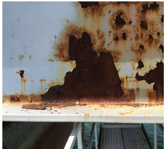
PHOTO 2 Description Span #12, girder #2 approximately 5' from bent #11 has corrosion with pitting to exterior web.
