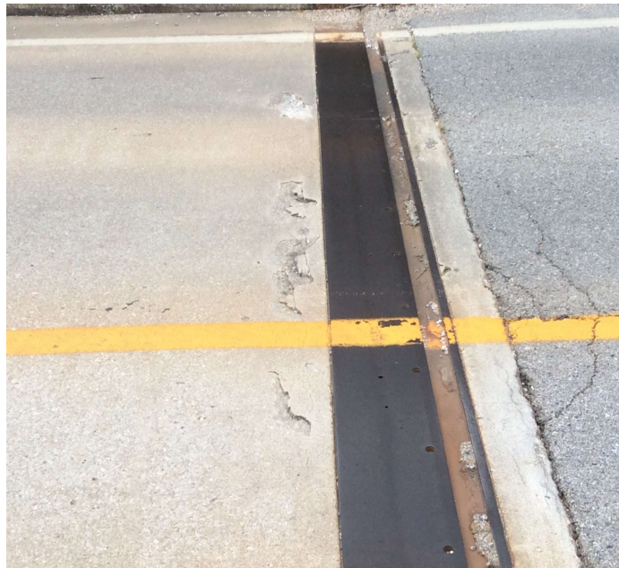
PHOTO 1 Description Spalling adjacent to abutment #1 sliding plate assembly.
