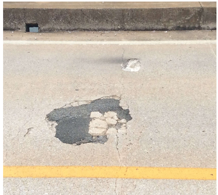
PHOTO 6 Description Deck spalling typical.
