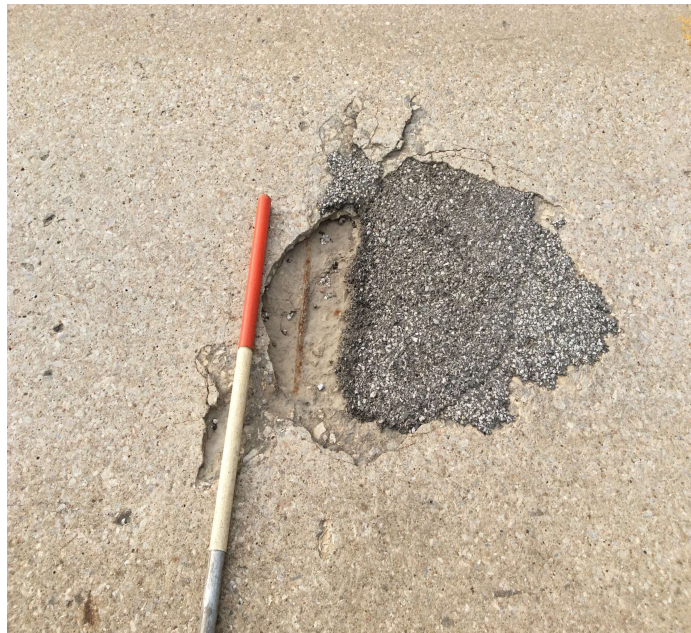
PHOTO 3 Description Deck spalling typical.
