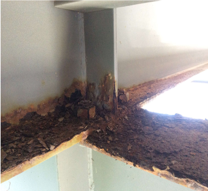
PHOTO 3 Description Corrosion at stringer / floorbeam connection.
