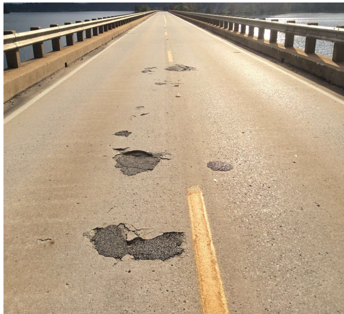
PHOTO 4 Description Deck spalling typical.
