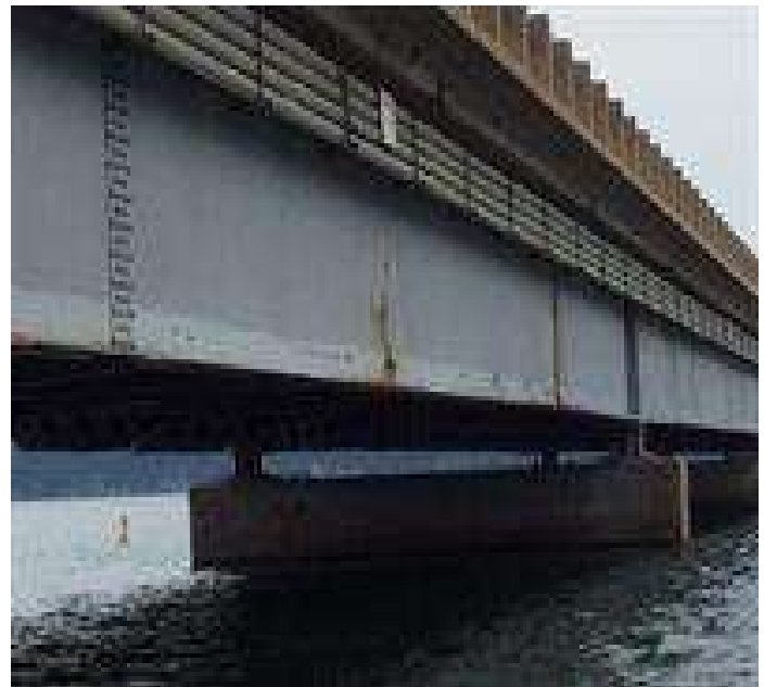
PHOTO 2 Description span #2 corrosion with minor section loss
