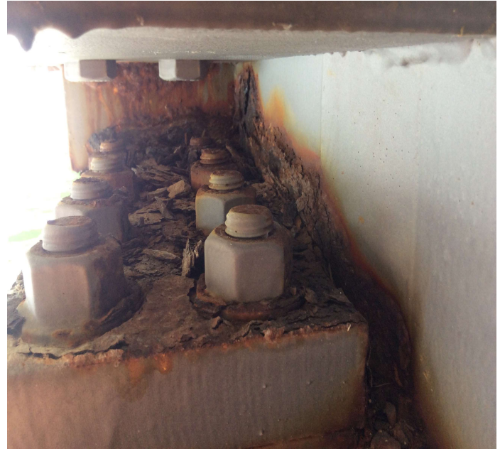
PHOTO 5 Description Corrosion to girder adjacent to pin and hanger assembly.
