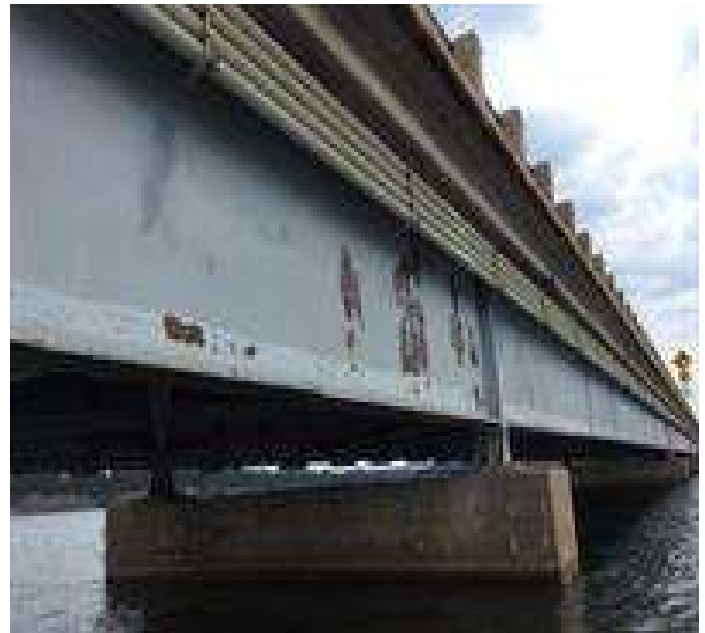
PHOTO 5 Description Paint condition right side
