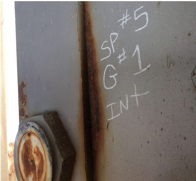
PHOTO 3 Description Corrosion with pack rust to pin and hanger assemblies.
