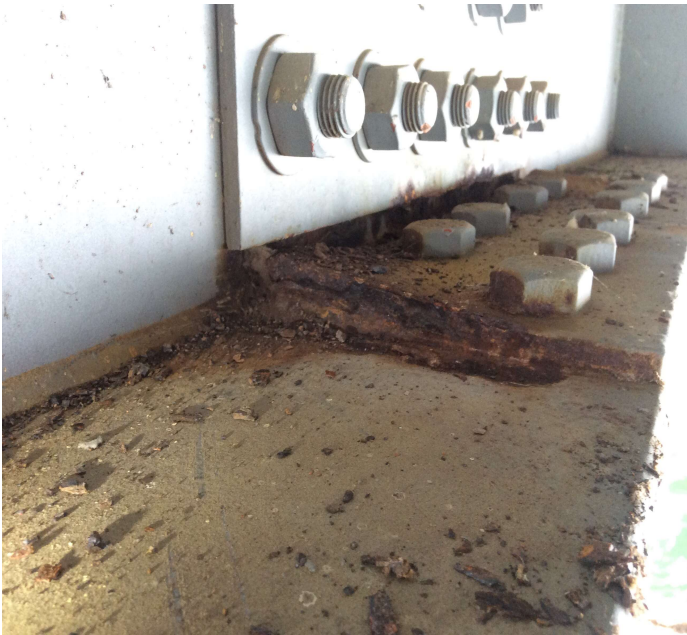
PHOTO 3 Description Pack rust with out-of-plane bending to connection plate.
